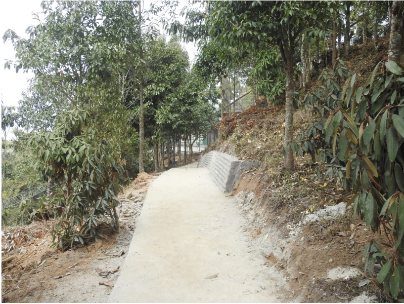
Fig: Construction of cement concrete pathway at Topkeydara
