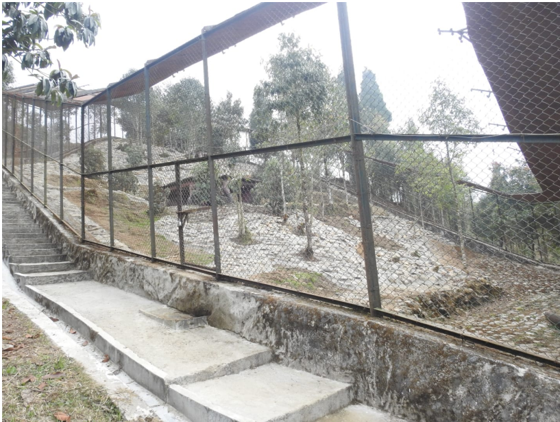
Fig: Enrichment of snow leopard enclosure by rubble masonry at Topkeydara
